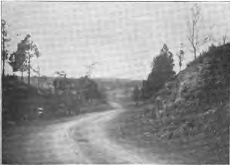
Marshall's Corner and Woodsville road, Mercer Co., after improvement.
